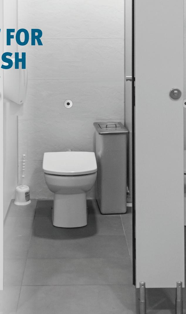
**Hygiene Flush:** To maximize hygiene, this product is equipped with a 24 hours duty flush. The flush takes place after 24 hours of non use have passed. Prevents the trap seal from drying out, possible freezing of pipes, and gets rid of potential bacteria in stuck water. This function can be disabled using the remote control.
